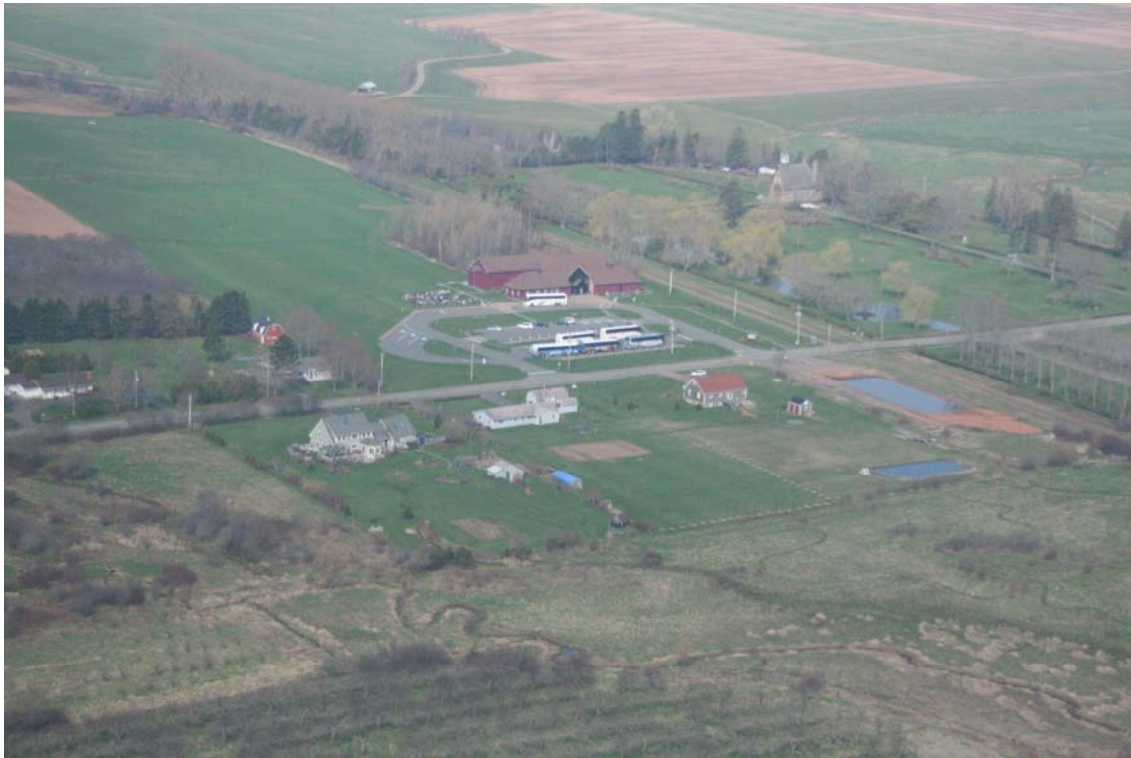
Figure 11: Aerial view of Grand-Pré National Historic Site of Canada. The visitor centre (large red building) was completed in 2003 and offers visitor services and interpretation programs to tens of thousands of visitors annually. It is the primary cultural attraction in the community.
