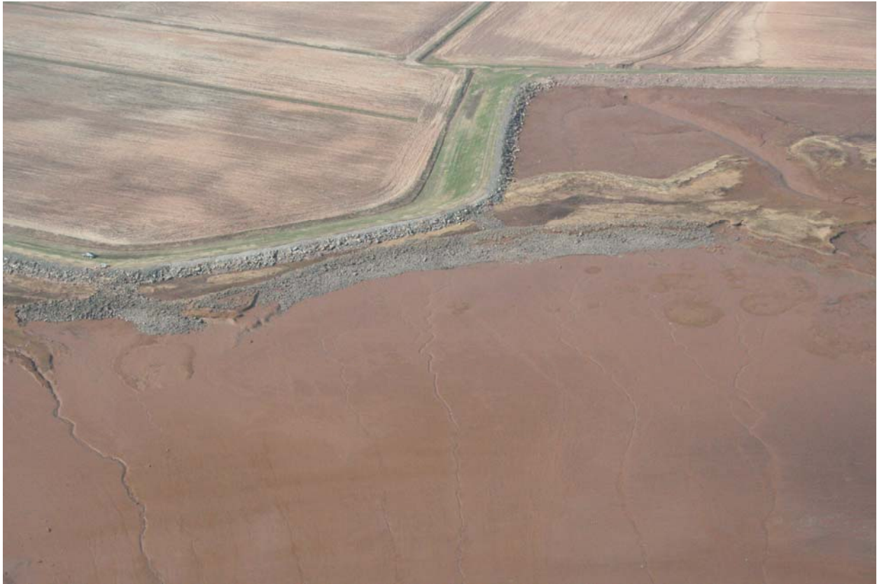
Figure 10: Coastal erosion is a constant pressure on the dykes. Above is a picture of the east facing dykes at extreme low tide. Top right corner: remnants of the salt marsh. In the middle: rock facing on the dykes and breakwater. Both have been weakened by the constant pressure.
